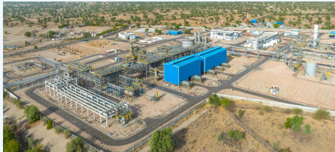
Rajasthan: Raageshwari Gas Terminal
