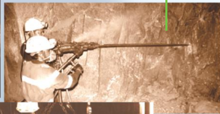
Drilling by hand-held hammer
