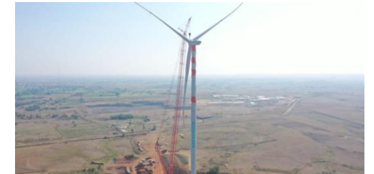
1st wind turbine installed
