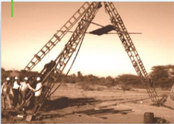
Conventional drill rig
