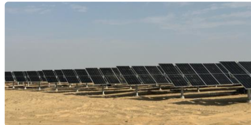
Modules installed at site
