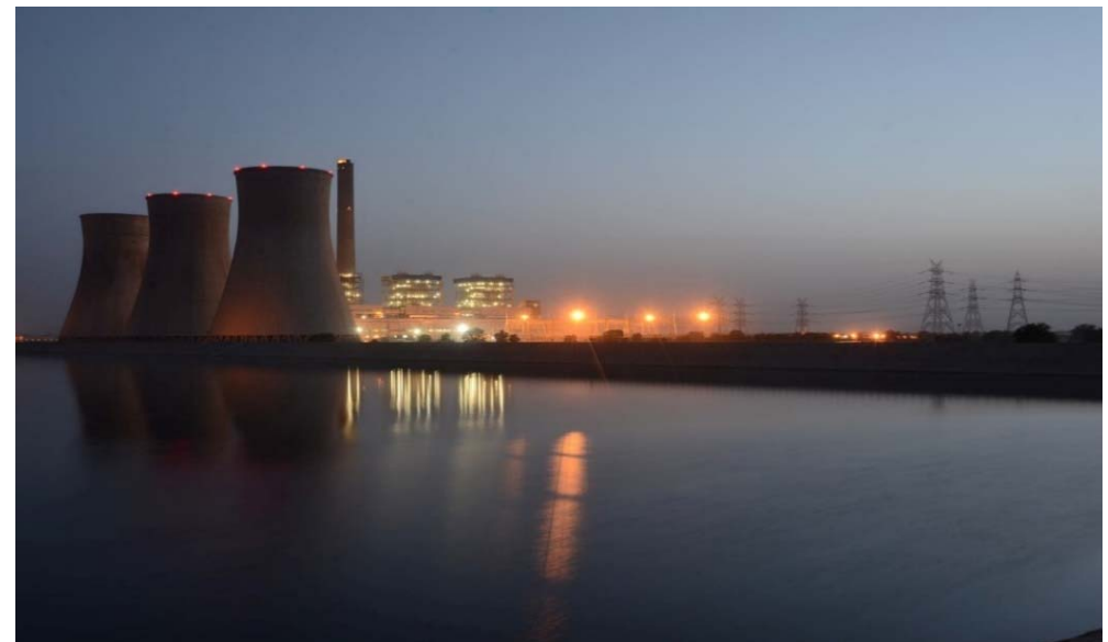
Talwandi Sabo Power Plant
