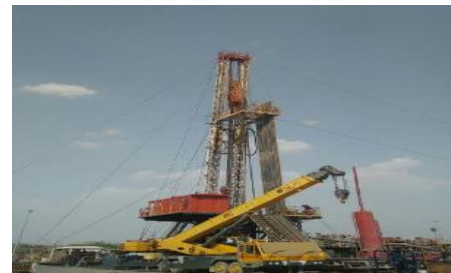
Drilling Rig at Mangala
