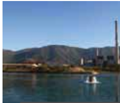
Raw water pond, VAL Lanjigarh
