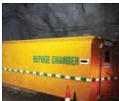
Refuge chamber in Rampura Agucha underground mine
