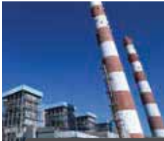
View of our SEL operations
