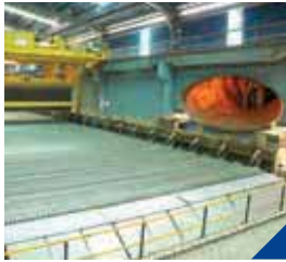
Cell house at Dariba zinc smelter, HZL
