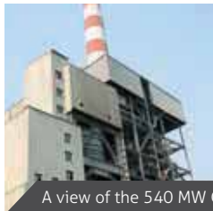
A view of the 540 MW CPP, BALCO
