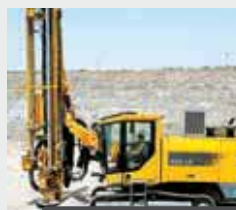
Operator operating driller at underground Rampura Agucha lead-zinc mine, HZL
