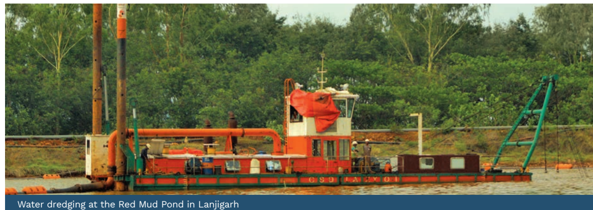
Water dredging at the Red Mud Pond in Lanjigarh
