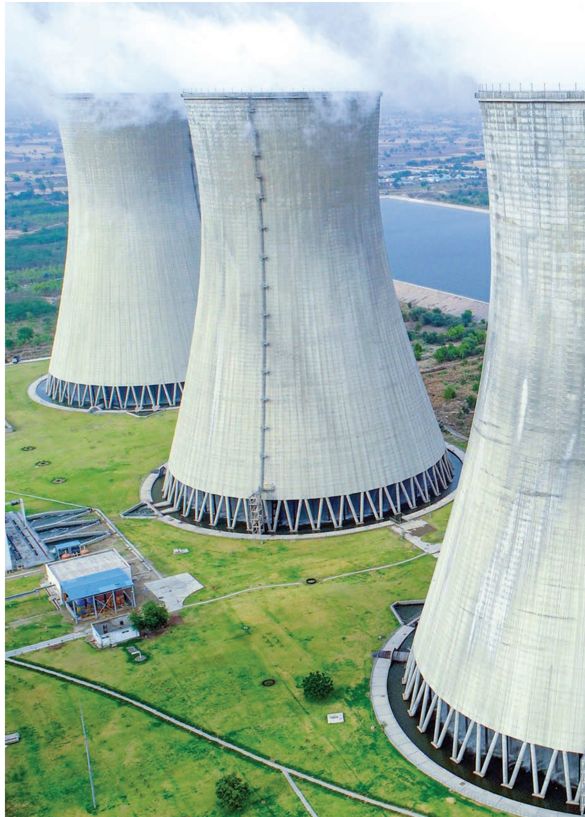
TSPL Power Plant
