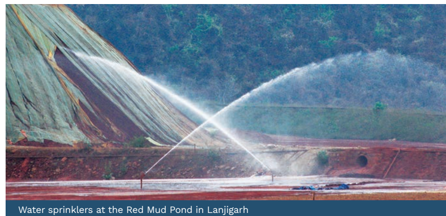
Water sprinklers at the Red Mud Pond in Lanjigarh
