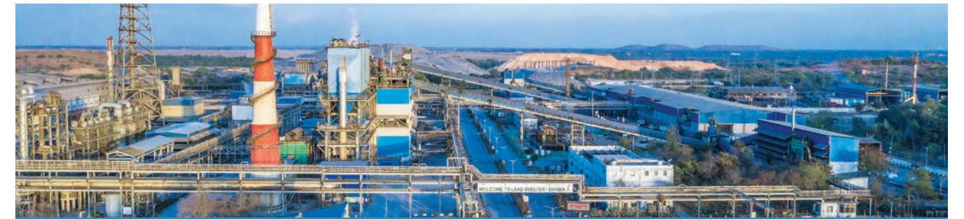
Dariba Lead Smelting Complex, HZL
