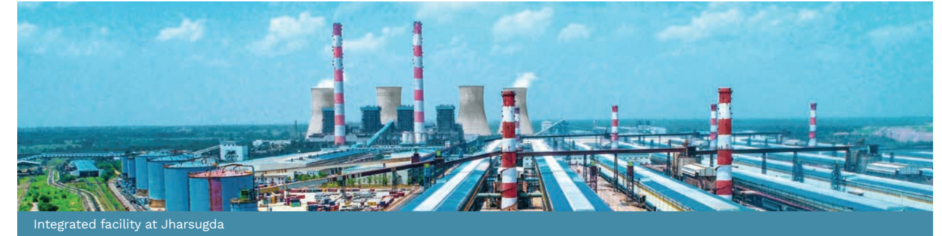
Integrated facility at Jharsuguda
