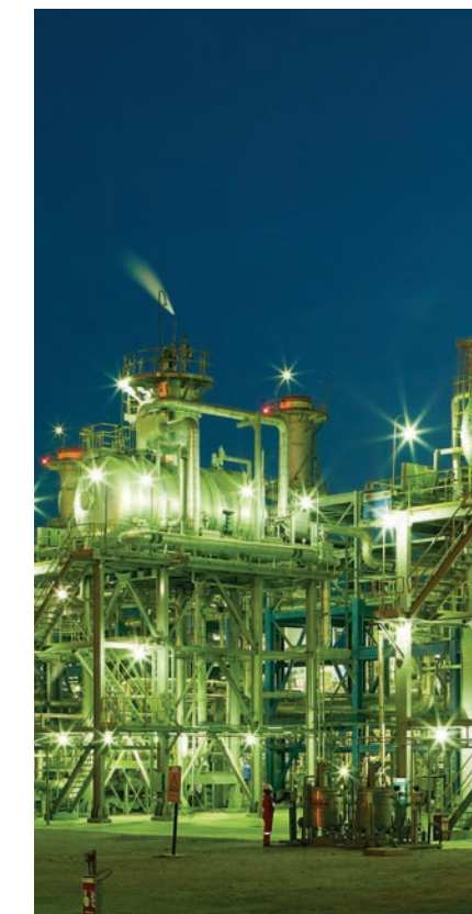
Mangala Processing Terminal at night, Barmer
