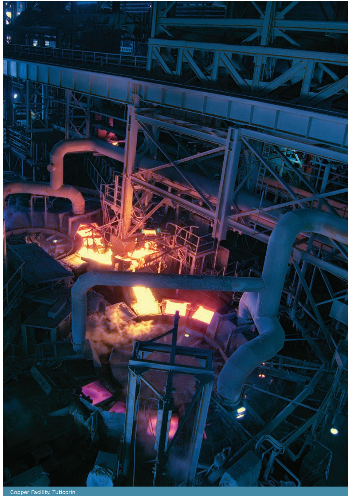
Copper Facility, Tuticorin
