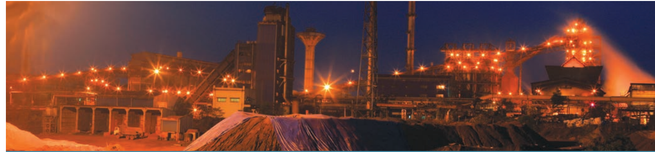
Value Added Business - Amona plant
