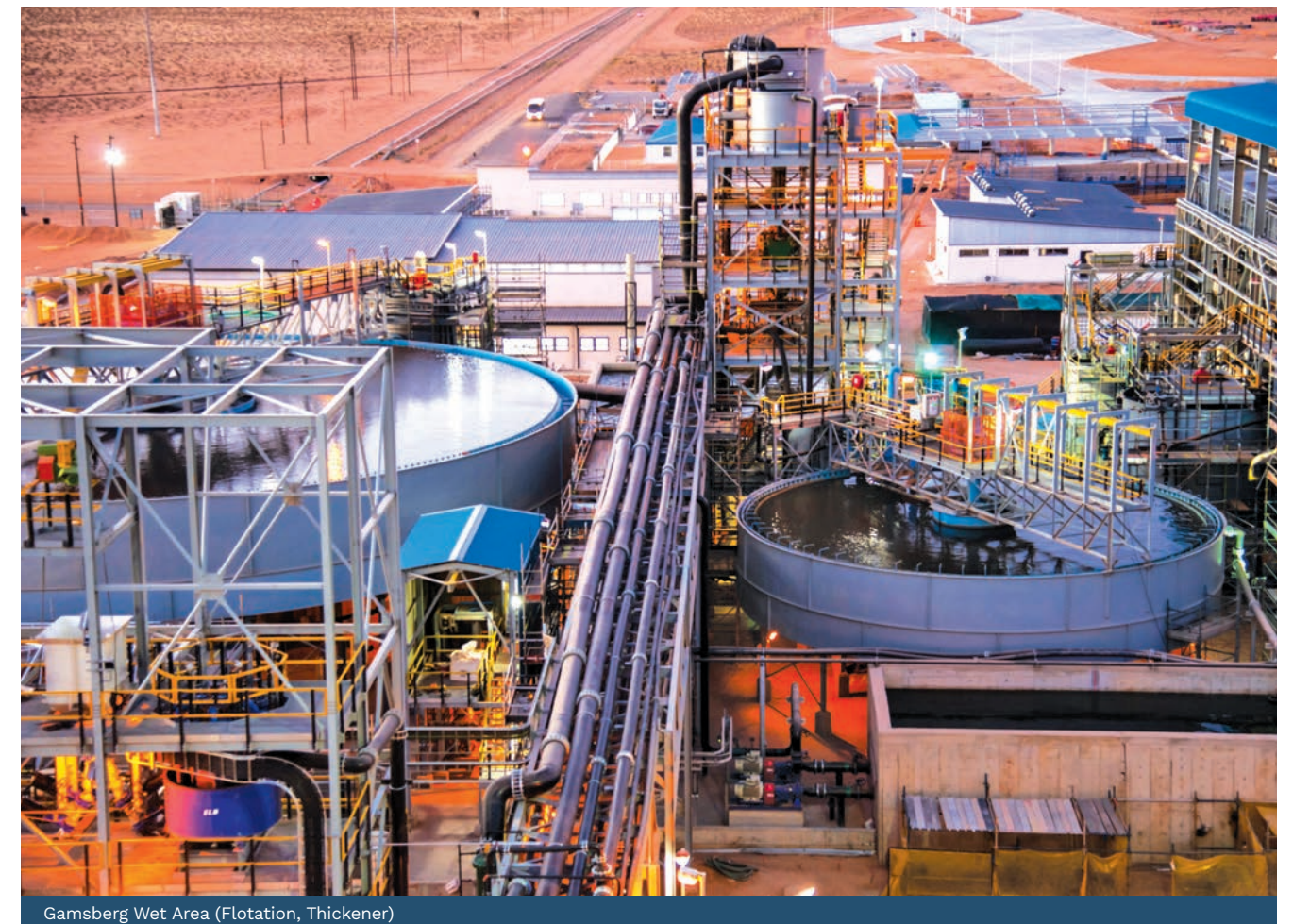
Gamsberg Wet Area (Flotation, Thickener)
