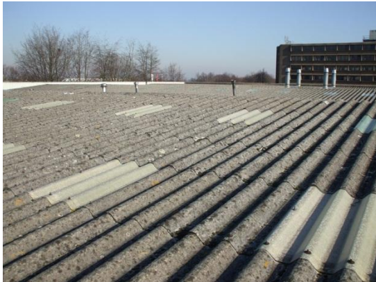
Example of fragile fibre cement sheeting where special precautions would be needed prior to commencing work.
