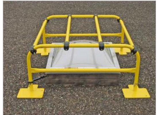
Falls through skylights are a common cause of fatalities during roof work. Temporary or permanent protection should therefore be used where there is a risk of fall.
