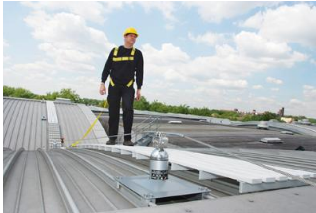
Example of crawling boards used together with horizontal lifeline and lanyard.
