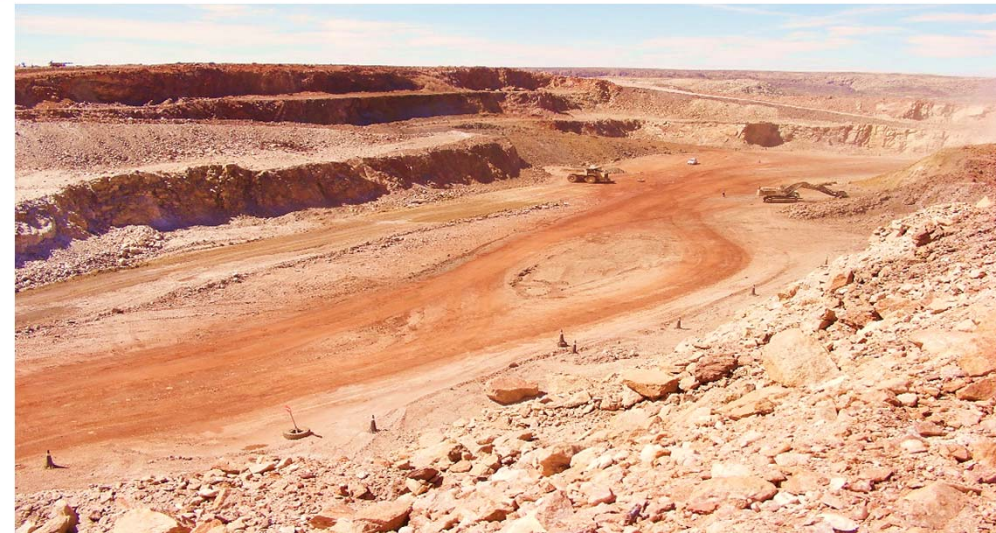
Gamsberg pre-start mining in progress (Dec 2016)
