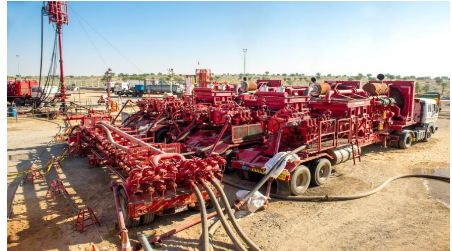
Fracking operations at RJ Block, Barmer, Rajasthan
