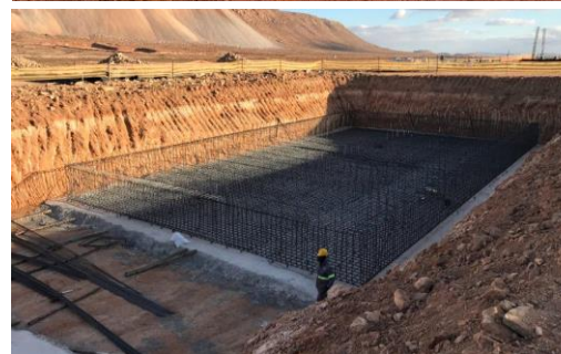
Ball Mill Foundation
