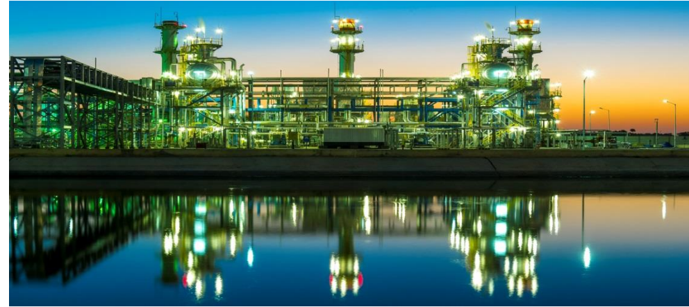
Rajasthan: Mangala Processing Terminal
