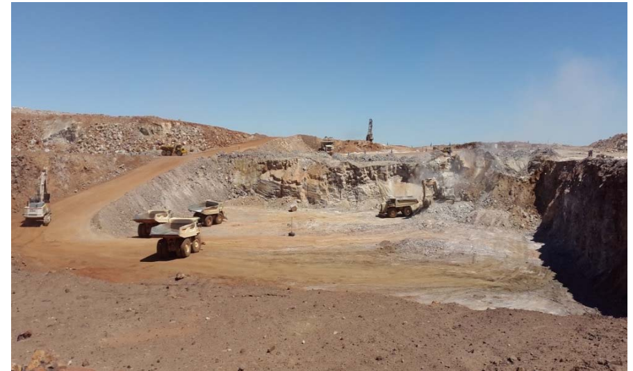
Pre-stripping at Gamsberg
