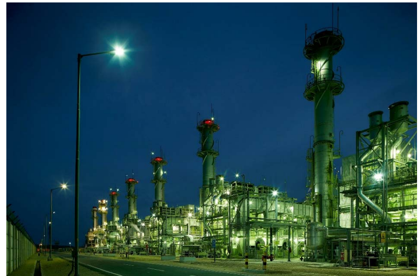
Rajasthan: Mangala Processing Terminal
