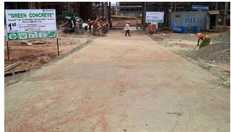
Road made of Cold-Setting Geopolymer Green Concrete at Lanjigarh
