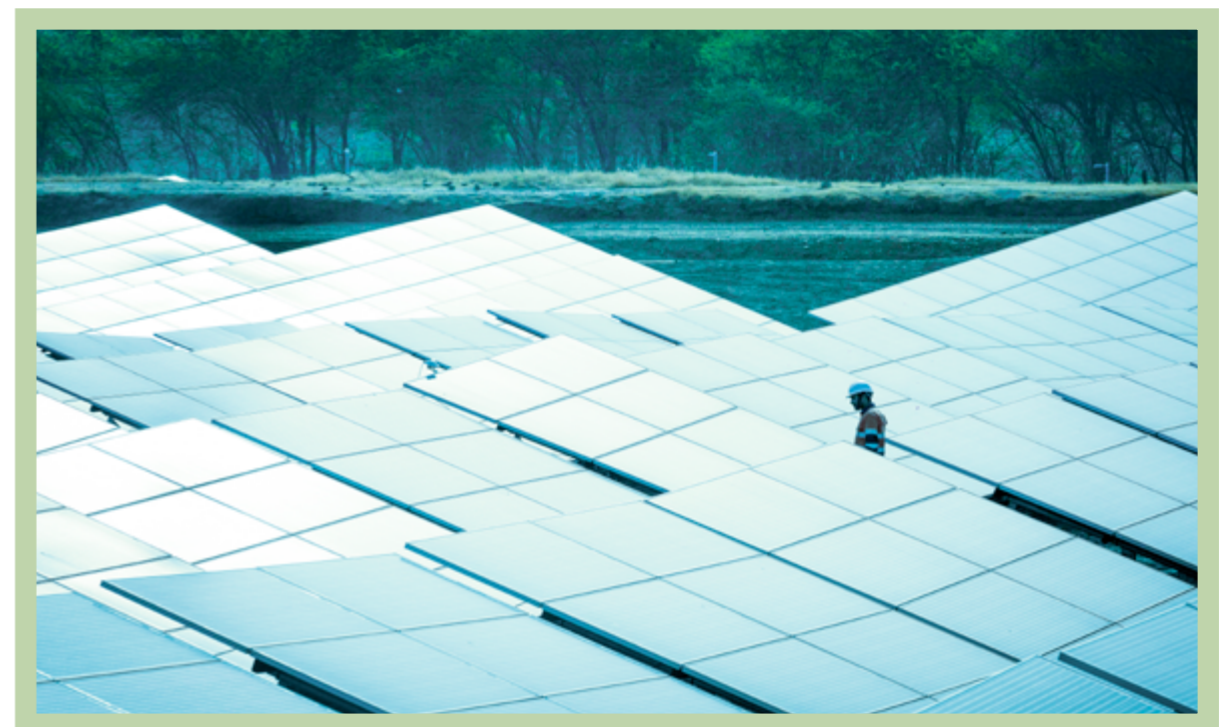
Solar Panels, HZL
